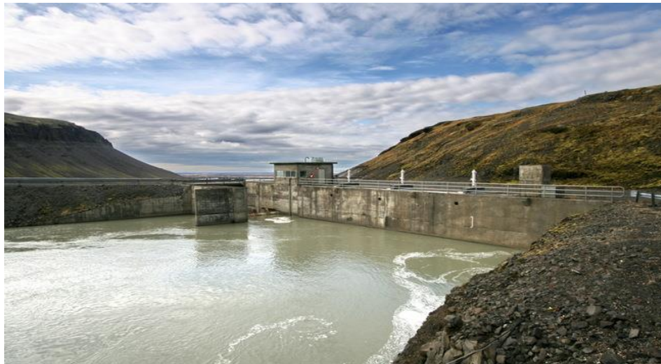
Fig. 3.Small hydroelectric plant - 1.2 MW, Ammassalik, Greenland
