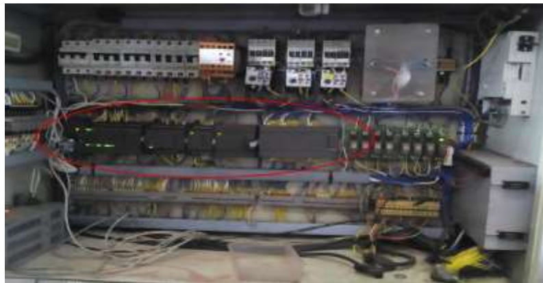
Fig.3.2: Example of a PLC application
