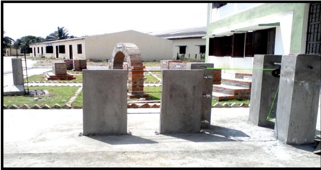
Fig.6.3: Shear wall portal frame
