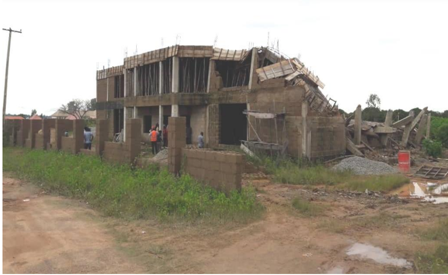
Plate 1: Inspection of the Collapsed Building and Physical Survey of the Soil
